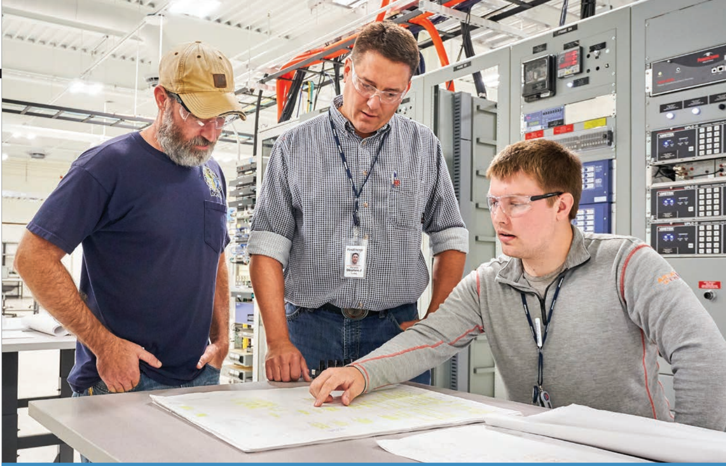
L to R: Brandon Dickriede, relay tester; Stephen Ciukaj, advanced relay technician; and Levi Propst, engineer III, work to develop new energy grid solutions at FirstEnergy's Center for Advanced Energy Technology in Akron, Ohio.
